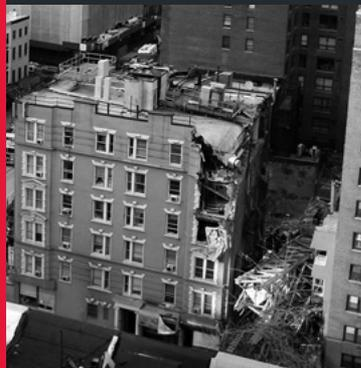
A large **construction crane** collapsed in Manhattan on March 15th, 2008, killing seven people and hospitalizing several others in critical condition. New York City's Department of Buildings found that the contractors in charge of the crane were reckless in regard to rigging techniques and that one of the department's inspectors had filed a false inspection report.
